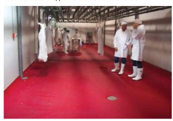
ROXSET SE1 is ideal for wet processing zones such as food manufacturing, food preparation areas and chemical processing plants. ROXSET SE delivers an easy to clean and sterilize anti slip surface, which is heat resistant to 120c and provides thermal protection at -40c. In the cold room areas ROXSET SE4 was applied. The seamless flooring also ensured compliance with all the requirements of HACCP, AQIS & BRC certification. Wall-to-Floor coving installed at 100ml to provide a monolithic surface.
