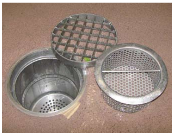
Self draining, continuous smooth surface and easy clean, replaceable components of a Blucher Industrial Drain.
