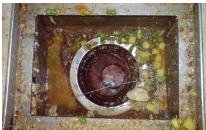
A high maintenance floor drain – Substantial product build-up, sharp corners and difficult to clean surfaces increase the risk for major bacteria issues.
