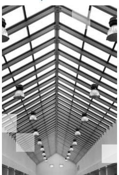
**Highbay lights** ('highbays') are mounted close to the ceiling in areas with high ceilings such as in warehouses and large processing areas. They are mounted using a pendant chain or cable or are fixed directly to a ceiling structure or beam.
